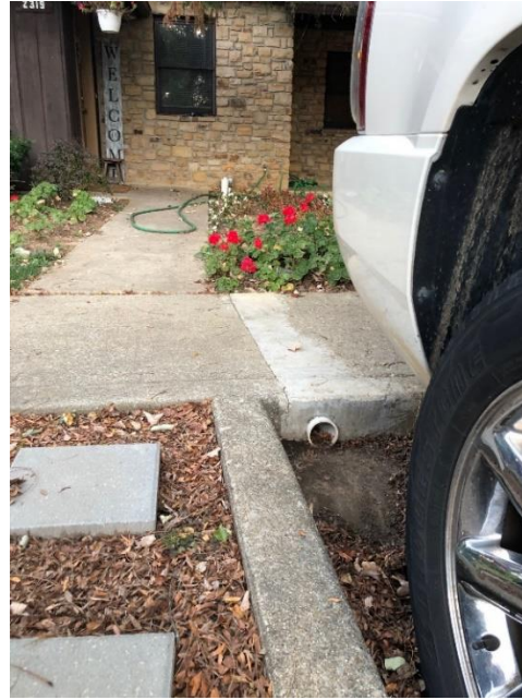
Drain similar to the community wide drainage project
