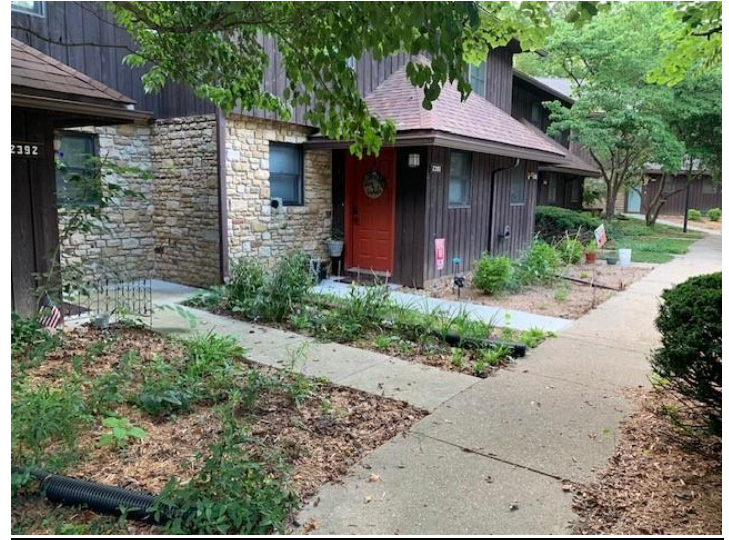
Building 2, part of phase 1 of the community drainage repair
