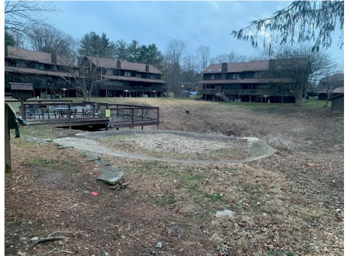
Stormwater drainage area project that is top priority for 2024!!!
