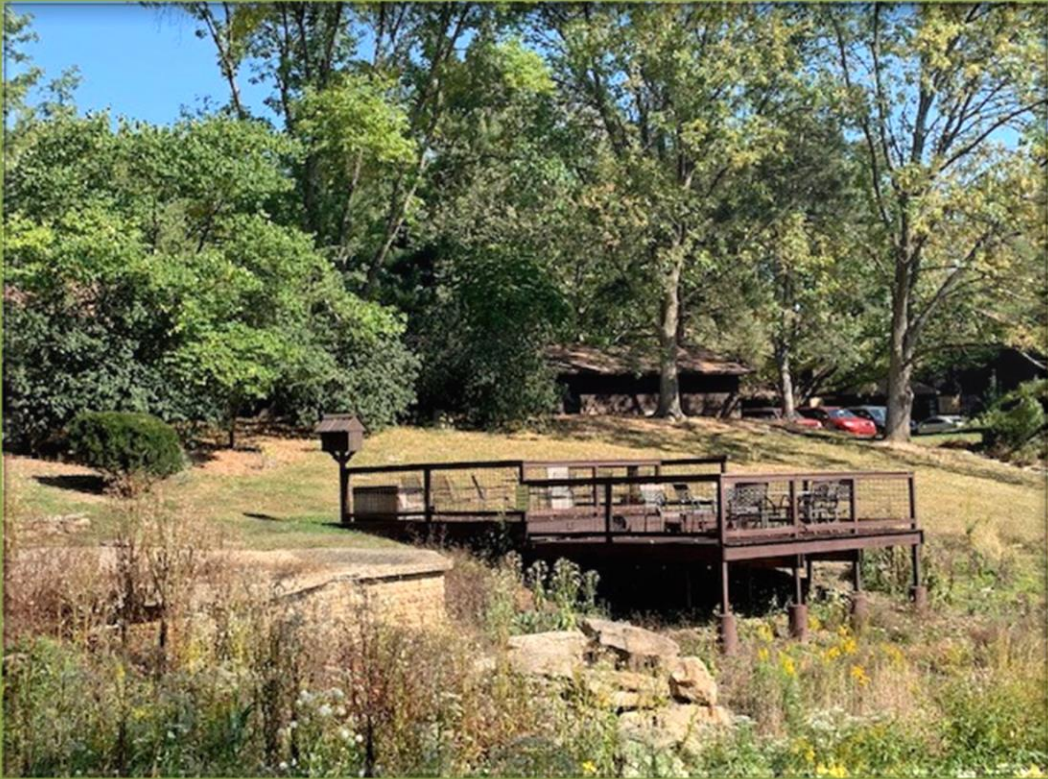
Modified Bioretention Area Deck
