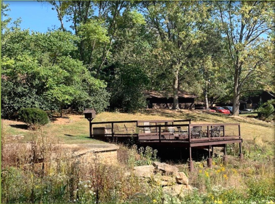
Modified Bioretention Area Deck
