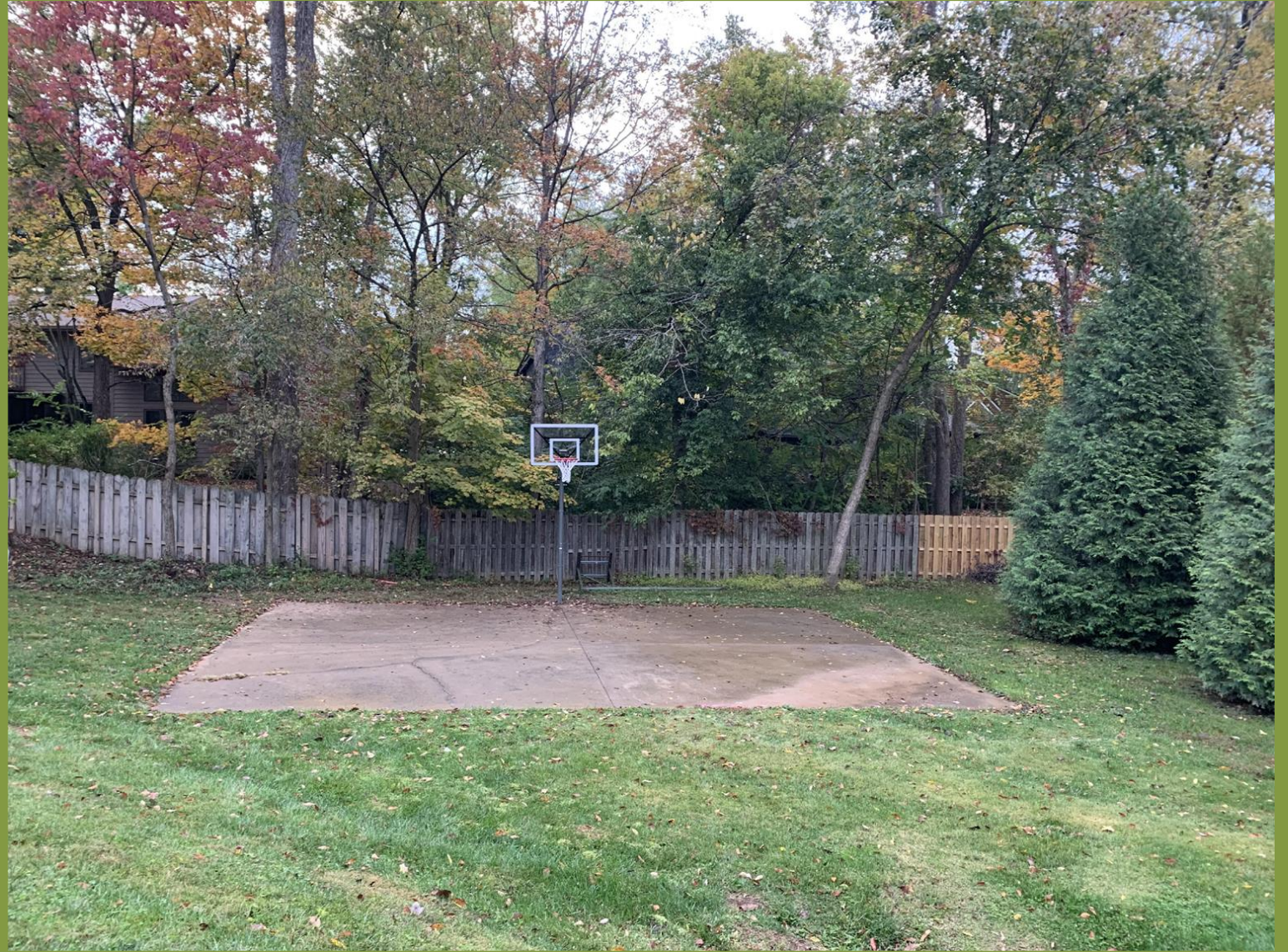
Basketball Court Repaired!
