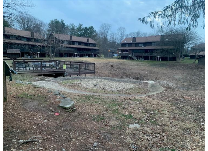
Obsolete pond area repair project for 2024!
