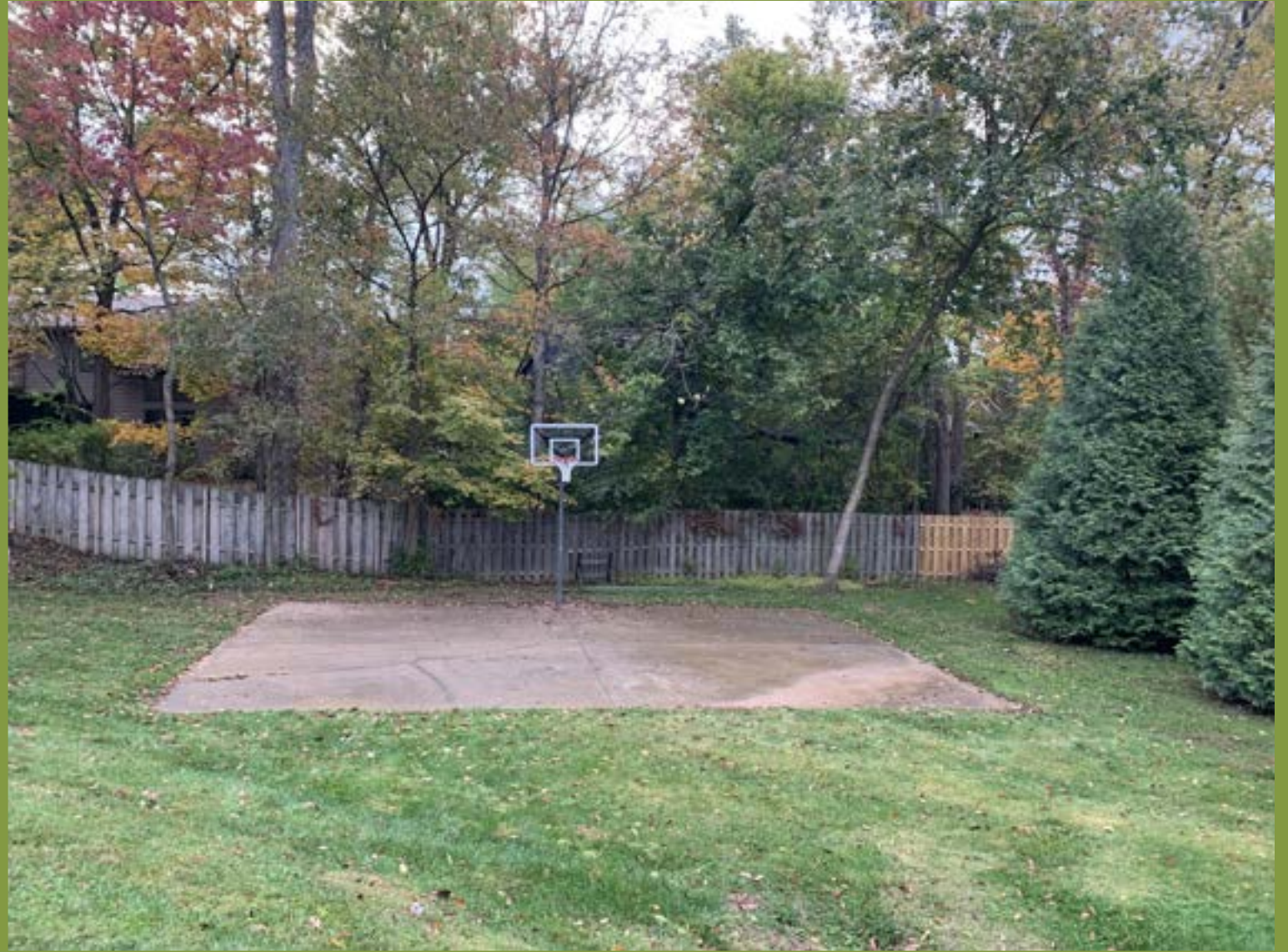
Basketball Court Repaired!
